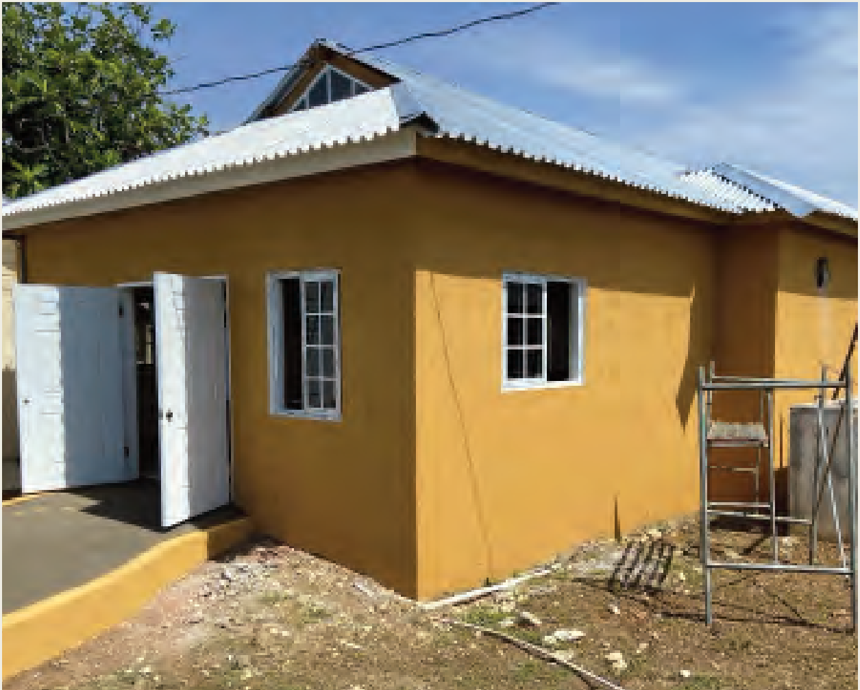
Newly constructed kitchen at the Hanover Infirmary.
