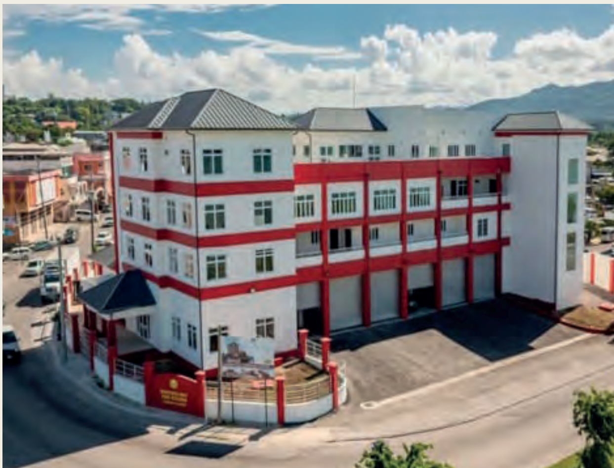
An aerial view of the Jamaica Fire Brigade Area 4 Headquarters, Montego Bay.
