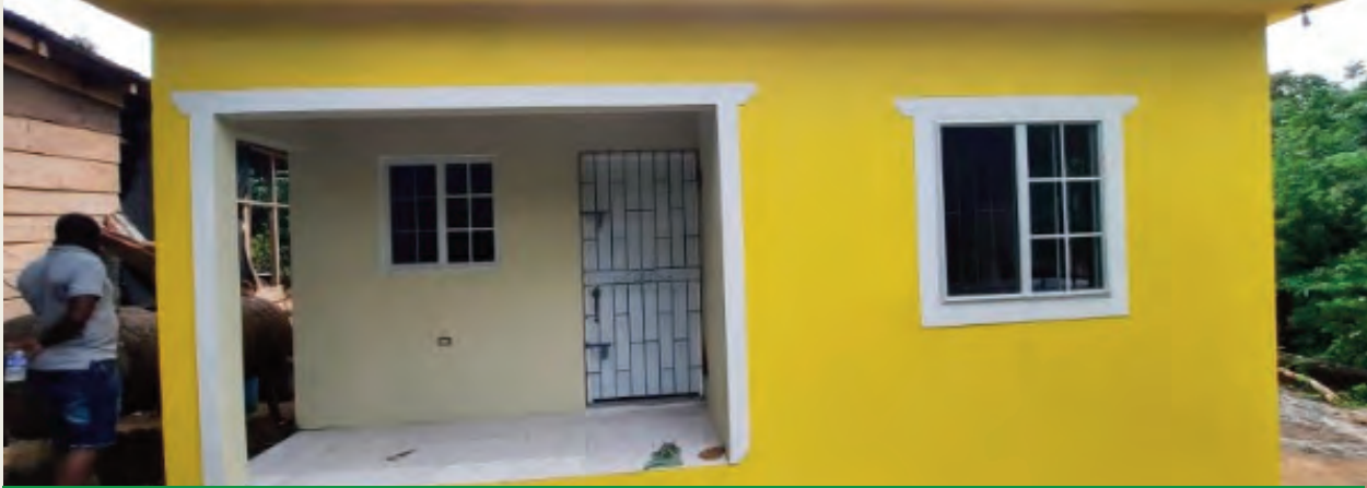
Completed Indigent House in St. Mary
